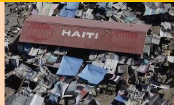
Earthquake in Haiti
